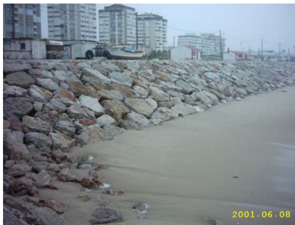
Figure 1.4 Groins consisting of rip-rap dumped rocks and well-placed rocks
