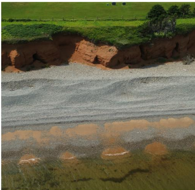
Figure 7.2.4 Beach nourishment of coarse sediments ( d_{50}\geq 40 mm) pebbles, Magdalen Island
