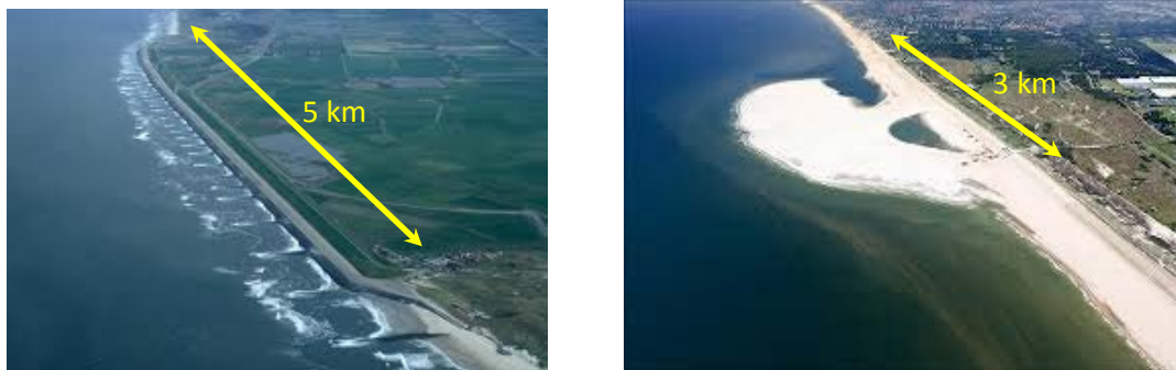
Figure 1.1 Land reclamation protected by seadike with groynes (left) and unprotected (right)
