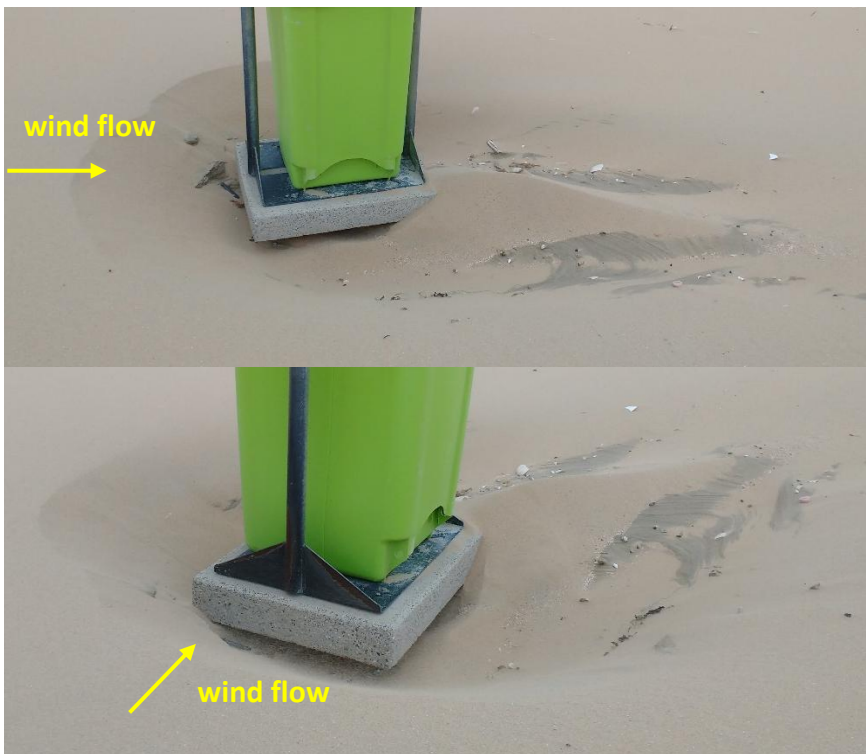
Figure 7.2.2 Scour around structure due to wind flow ( U_{wind} at 1 m \cong 10 m/s; U_{critical} \cong 5 m/s; d_{50} \cong 0.25 mm) (upper: side view; Lower: front view)
