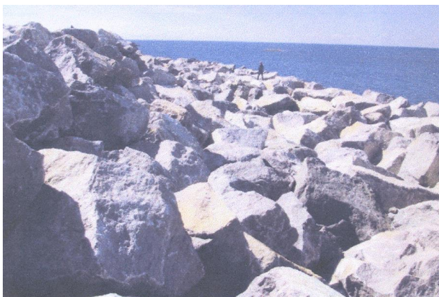
Figure 5.1.2 Icelandic-type berm breakers at Sirevag (Norway) and Husavik (NW Iceland)
