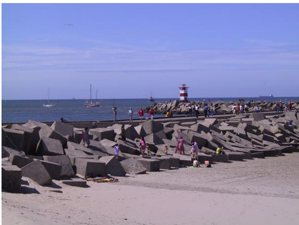
Figure 5.2.5 Breakwater of randomly placed cubes, fishery harbour Scheveningen, The Netherlands
