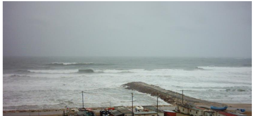
Figure 5.1.3 Coastal revetments and groins of orderly rocks at Caparica, South of Lisbon, Portugal
