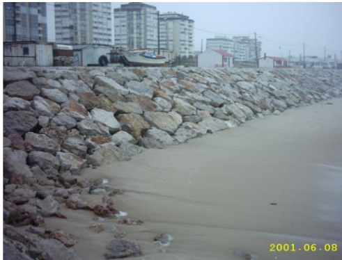
Figure 5.1.3 Coastal revetments and groins of orderly rocks at Caparica, South of Lisbon, Portugal
