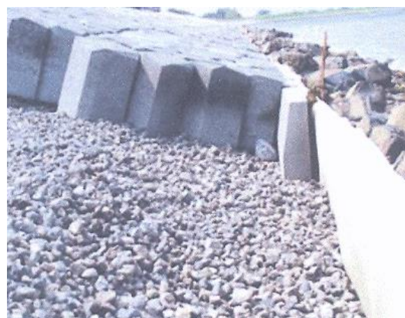
Figure 4.1.3 Armouring made of concrete blocks (Basalton) on thin granular levelling layer and geotextile
