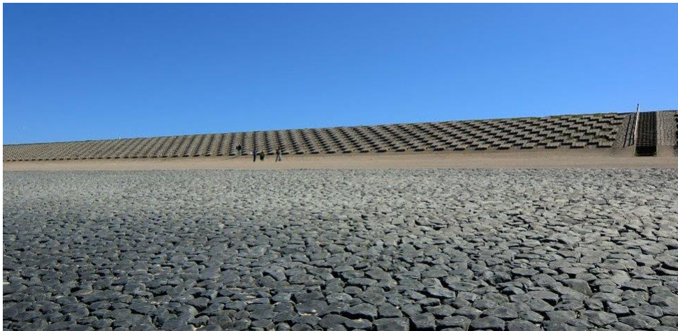
Figure 4.1.1 Seadike between Camperduin and Petten, The Netherlands (Crest = 12.8 m above MSL, Berm at 5.5 m above MSL, Slopes between 1 to 4 and 1 to 8)
