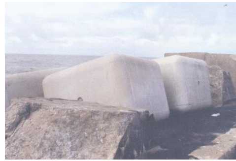
Figure 5.2.4 Desintegrated concrete cubes (left) and new cubes (right); IJmuiden, The Netherlands
