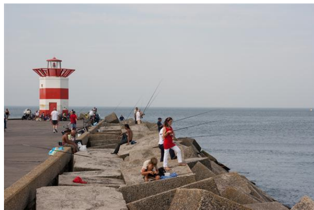
Figure 5.2.5 Breakwater of randomly placed cubes, fishery harbour Scheveningen, The Netherlands
