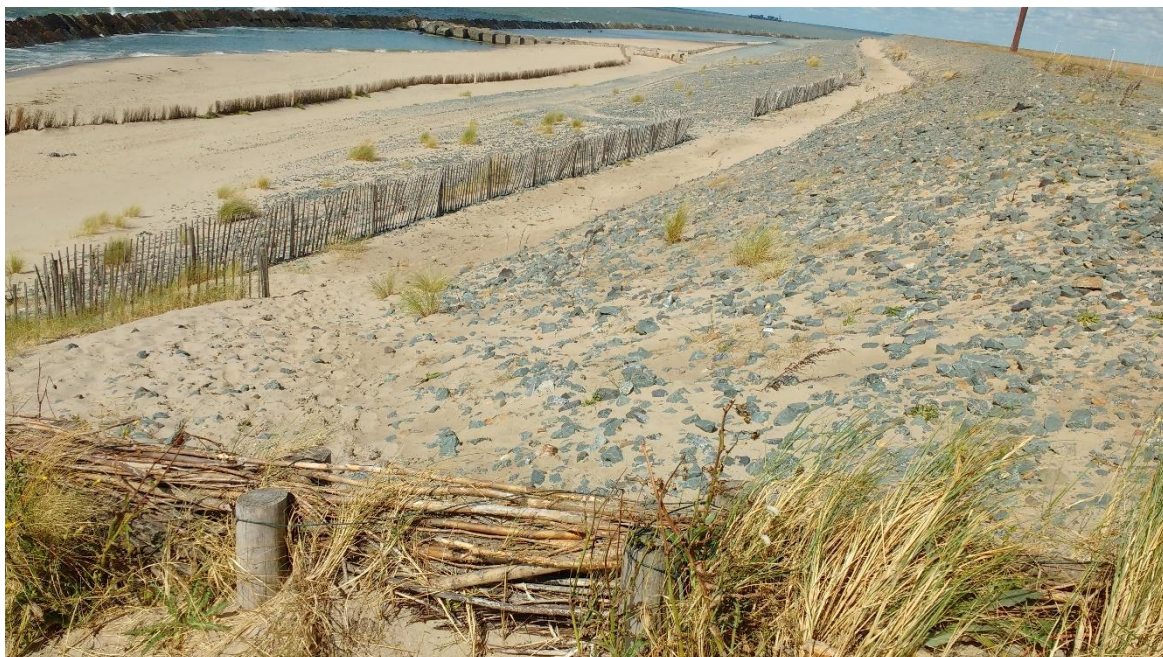
Figure 4.1.7B Sea defence of Maasvlakte 2 at transition from sandy beach to hard defence (August 2018) Upper: sand beach; Middle and Lower: hard sea defence with concrete cubes and cobbles
