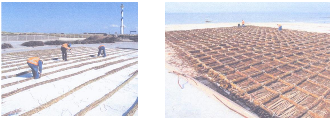
Figure 6.2.3 Preparation of geotextile for massive breakwater
