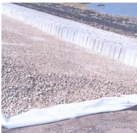
Figure 4.1.3 Armouring made of concrete blocks (Basalton) on thin granular levelling layer and geotextile
