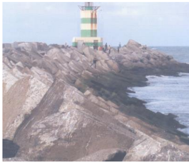
Figure 5.2.4 Desintegrated concrete cubes (left) and new cubes (right); IJmuiden, The Netherlands
