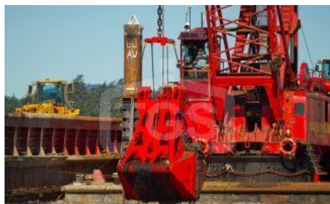
Figure 3.2 Grab dredging (The Grab Specialist; www.tgs-grabs.nl ; Almere, The Netherlands) Upper: open grabs with heavy mud spill during hoisting Lower: closed clamshell grabs (left:hydraulic for backhoe and Right: mechanical for crane)
